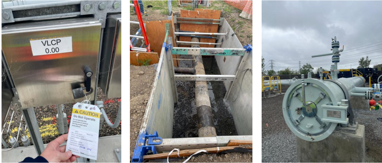
Figure 26: Representative Clearance Field Observations (Caution Tag (left), Replacement of Two Pipe Tees (middle), and Installation of a Pig Launcher (right))
