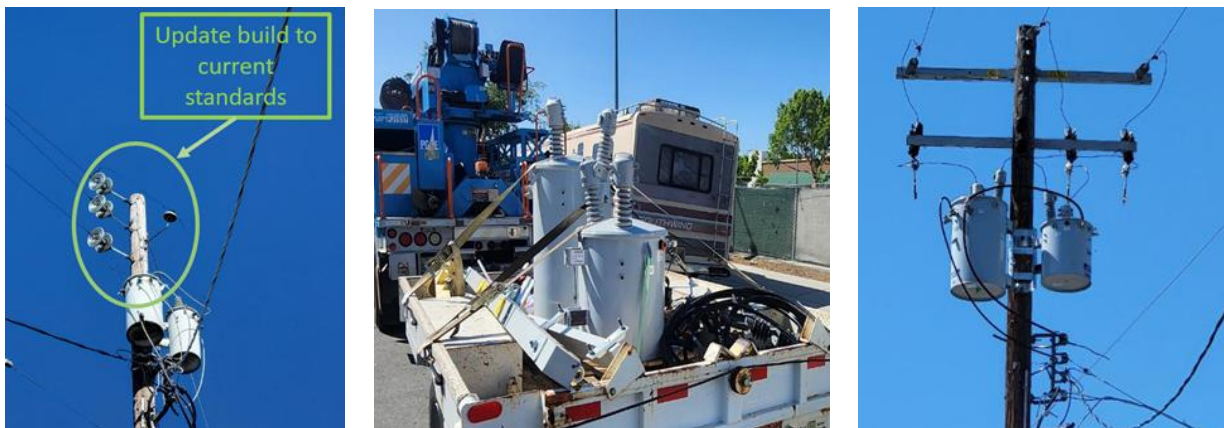
Figure 15: Representative Routine Maintenance Field Observations (A-Tag, Project Load-Out, and Completed Project)
