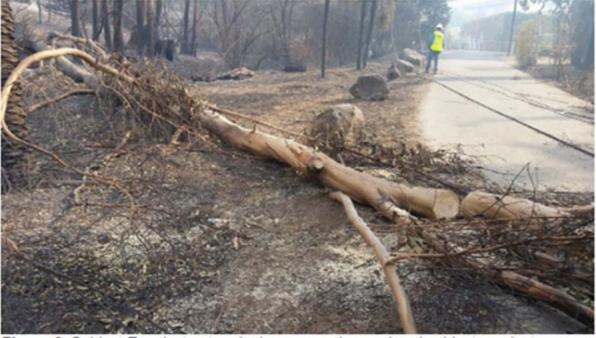
Figure 8. Subject Eucalyptus tree laying across the road and subject conductor spans. The tree was rooted in the top left corner of the image. (October 17, 2017)
