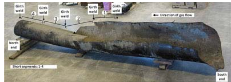
28-foot-long ruptured section of pipeline at laboratory facilities at the NTSB Training Center, Ashburn, VA
