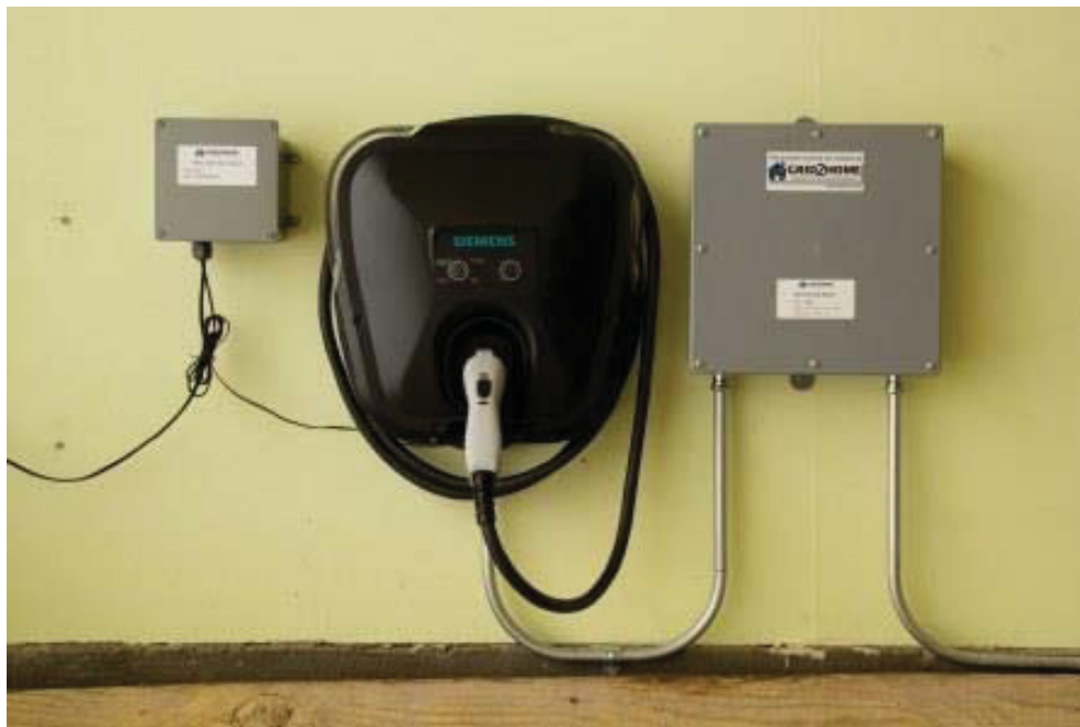
Figure 7- In this customer installation, the EVSE did not have enough space to place the Raspberry Pi (left) inside. The sub-meter on the right could be placed anywhere on the branch circuit, including next to the panel. This unit had a relay allowing only on/off capability (the small wire from the Raspberry Pi to the EVSE).
