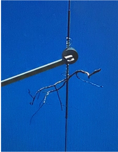
Figure 10: Image of Vegetation Hazard in Nevada County – Tree Limb Hanging on a Conductor
