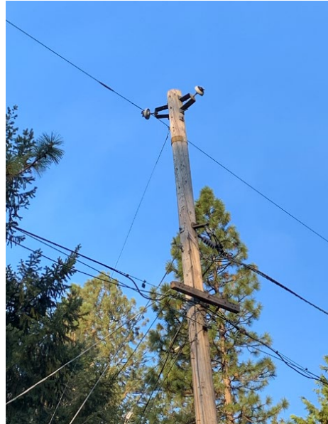
Figure 11: Image of Vegetation Related Damage in Butte County – Broken Insulator and Floating Conductor
