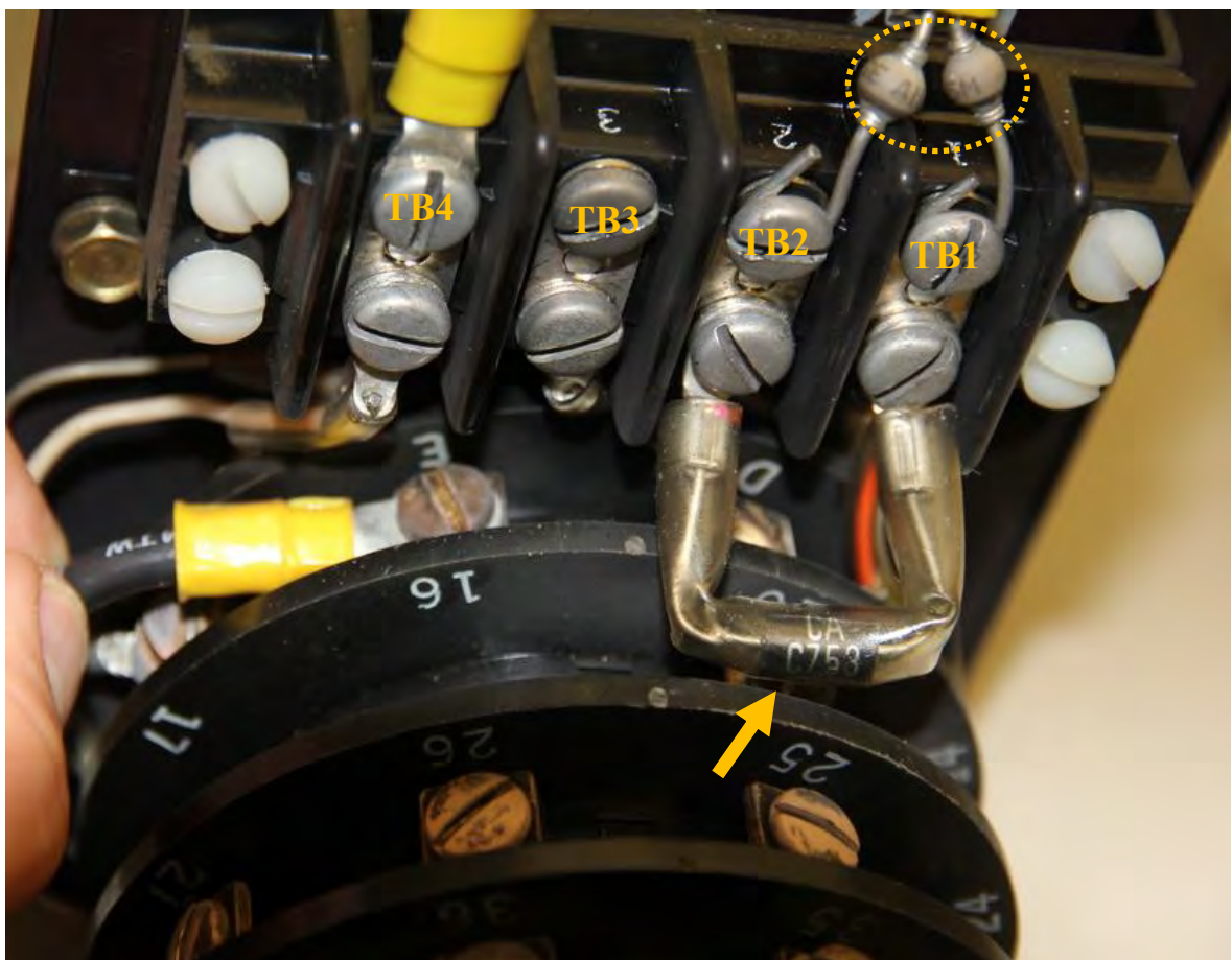
Figure 3. Two 600V fast recovery diodes (shown in yellow circle) and a bipolar diode (indicated by yellow arrow) attached to the incident switch terminals. The switch terminal points are marked TB1 to TB4.
