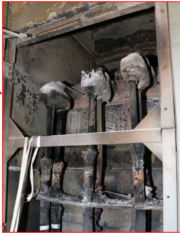
Figure 2. Damage at the “Tee tap” near the back of the incident cabinet.
