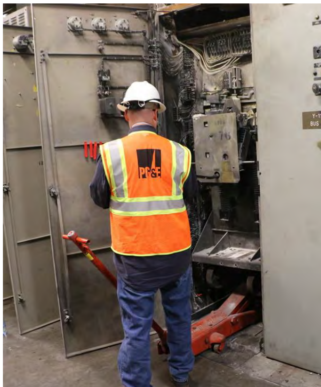
Figure 10. PG&E personnel were able to manually trip the incident breaker during the restoration process; this shows that the incident breaker did not operate at the time of the incident.
