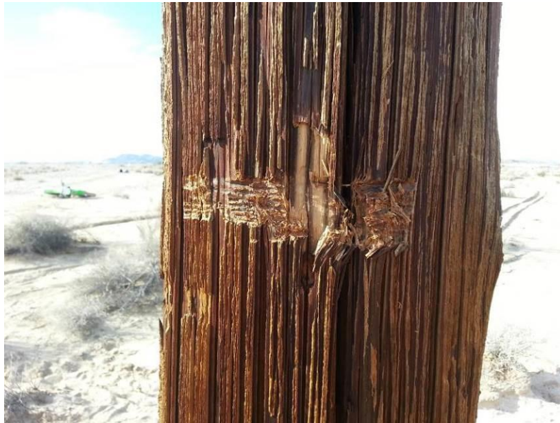
Figure 6: A scratch mark on Pole number 43502S.
