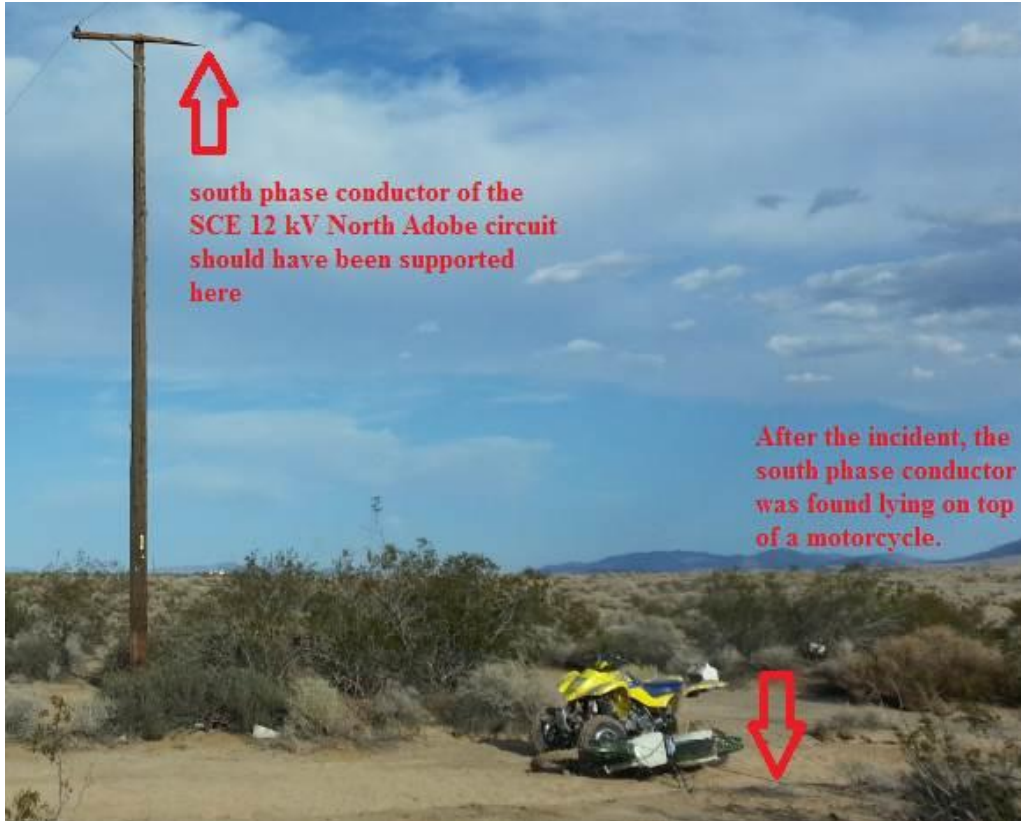
Figure 1. Image of the incident site showing the broken crossarm on Pole number 43502S.
