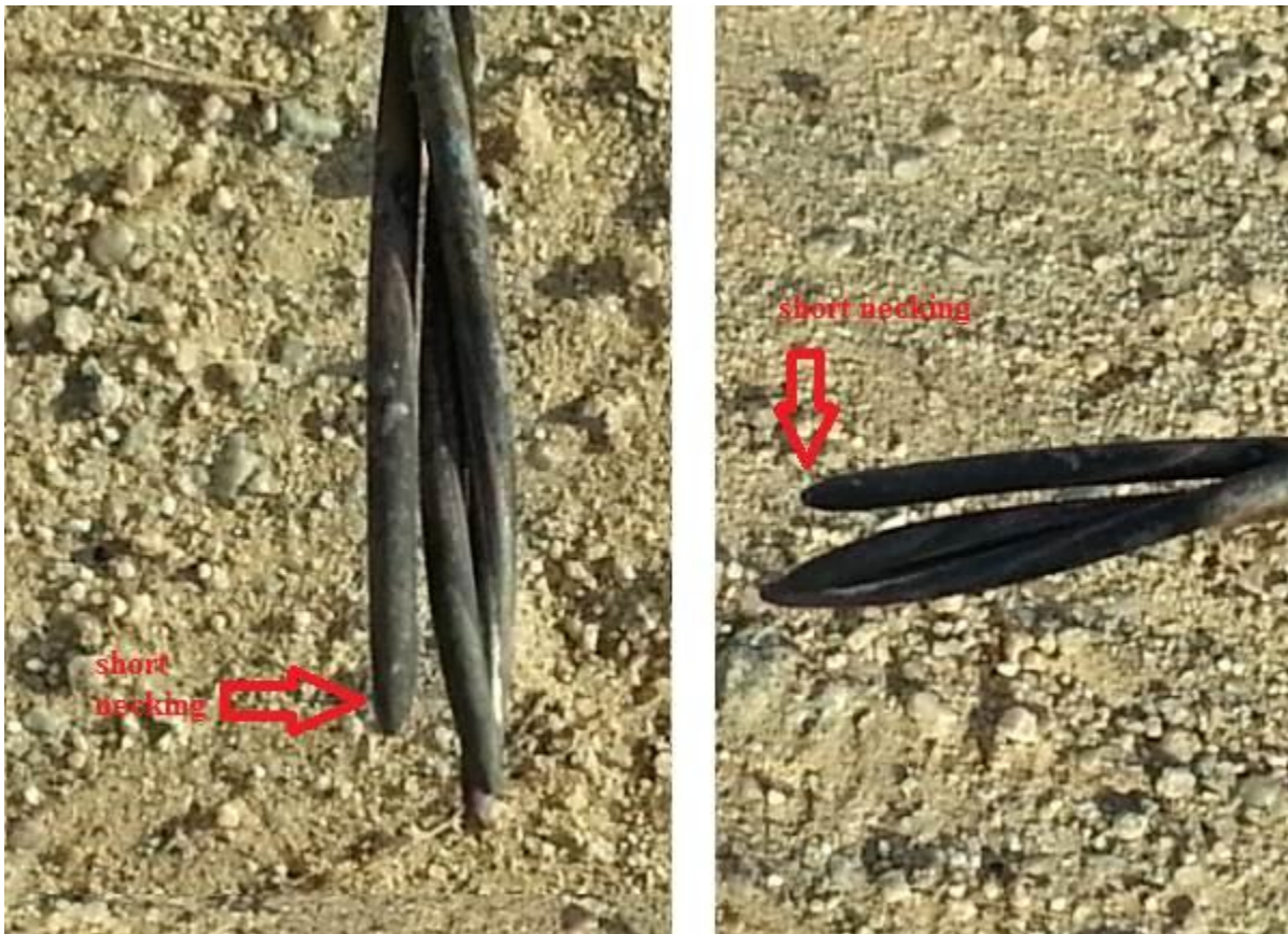
Figure 4. After the incident, the south phase conductor of the SCE 12 kV North Adobe circuit was found broken into two pieces and lying on the ground. The broken ends of the conductor exhibit short necking.
