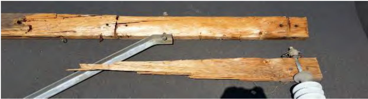
Figure B-2: The front face of Specimen 1 – right side close-up.
