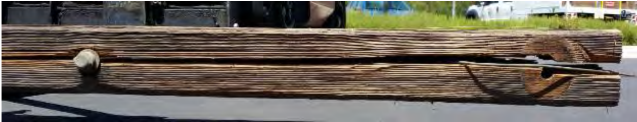
Figure B-11: The top face of Specimen 5 – right side close-up.
