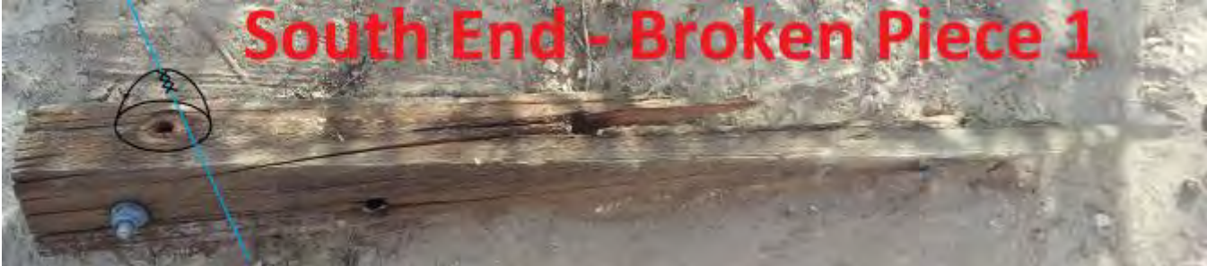
Figure A-4: "South End – Broken Piece 1" (photo 2/4) showing where the insulator would have been installed. Source: SED
