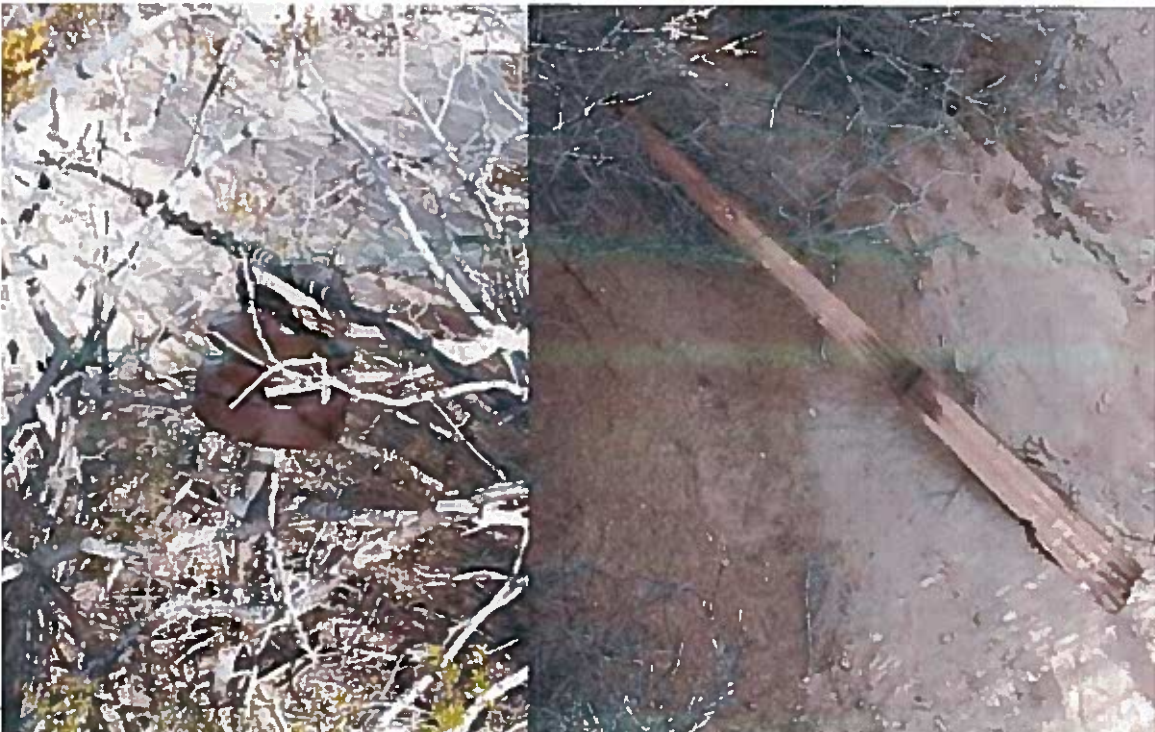
Figure 2. The left and right images show the insulator and crossarm that were supported on pole number 43502S.
