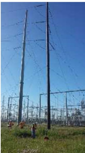
Figure 14 – New tubular steel poles replacement
