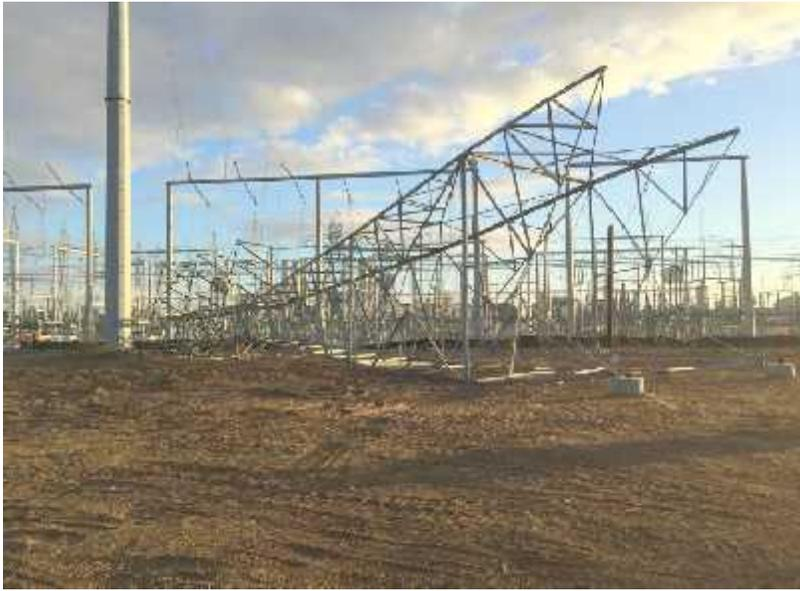
Figure 11 – Collapsed Tower 61/268
