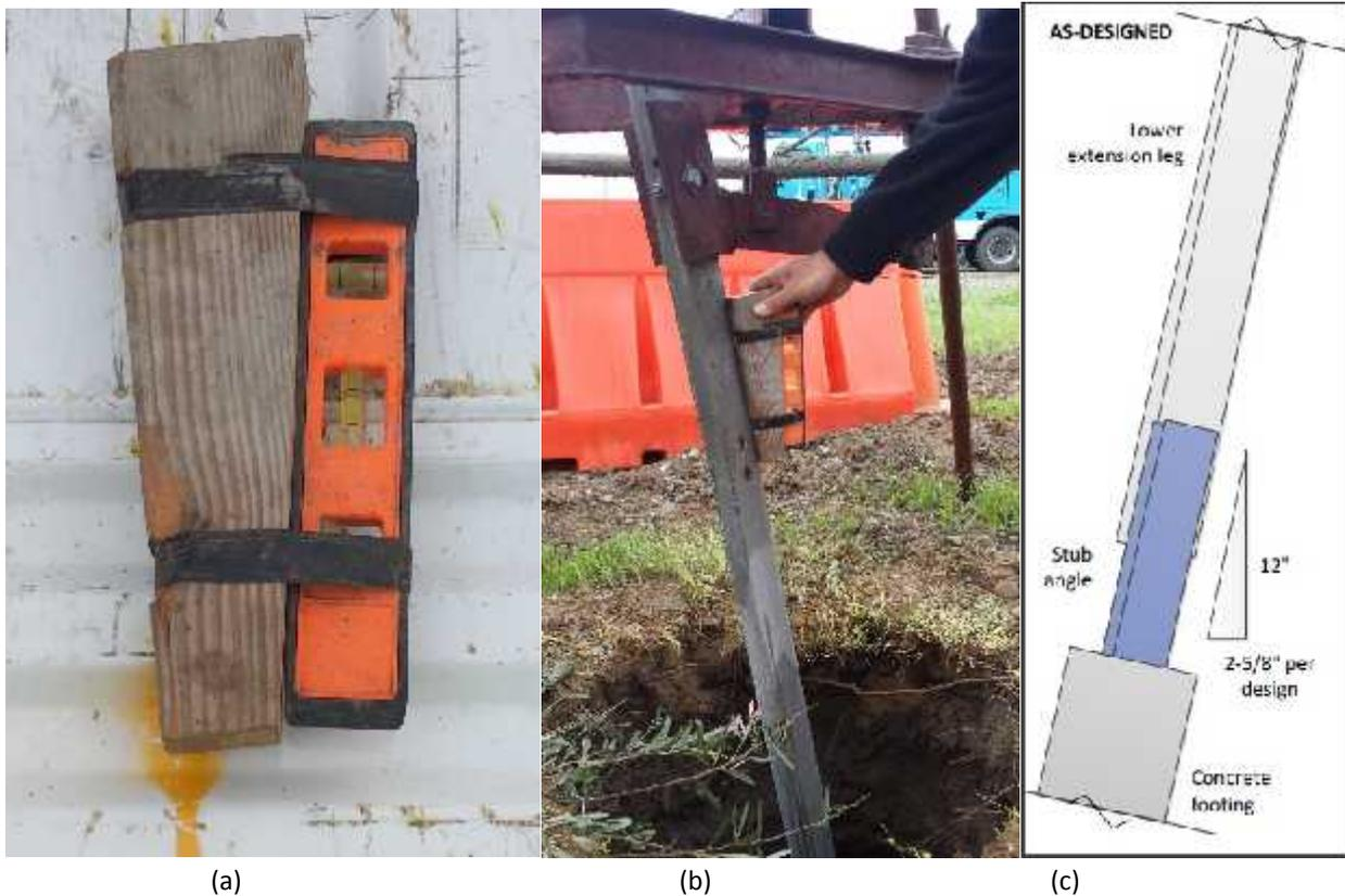
Figure 3: (a) Example of a batter board, (b) its use, (c) close-up of the bottom of a tower, detailing the concrete footing, stub angle, and tower leg.
