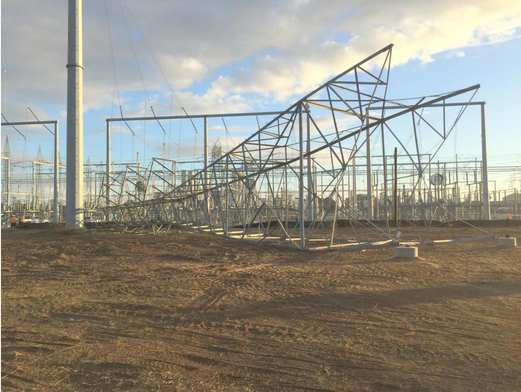
Figure 1: Moss Landing Tower Collapse Site Photo
