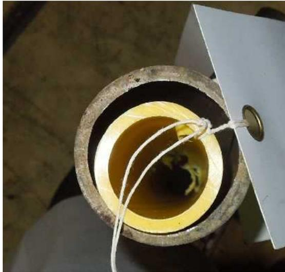
Figure 7: 1-1/4 plastic main inserted into 2 inch steel.
