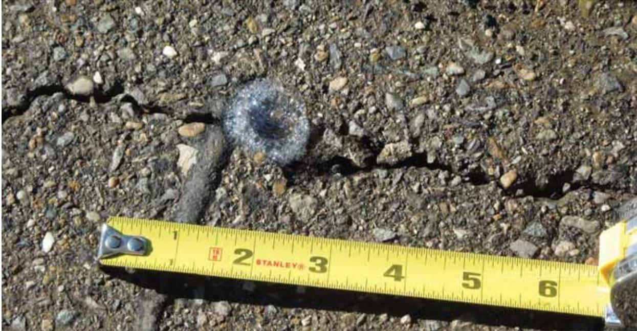
**Figure 7.** Air bubbles in driveway crack at [REDACTED]
