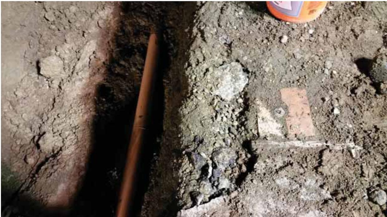
**Figure 9.** Exposed segment of main with the joint that was the source of the leak.
