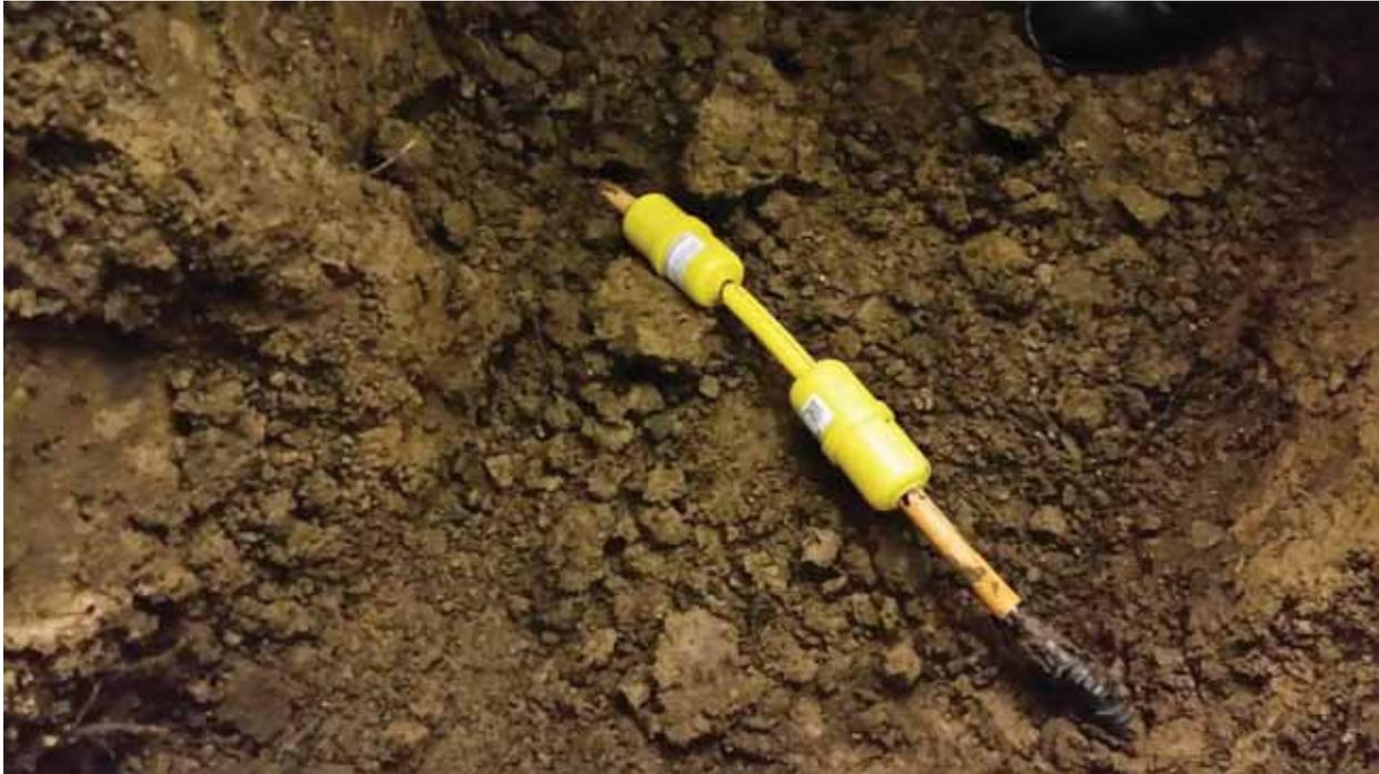
**Figure 6.** Severed service line repair at [REDACTED].
