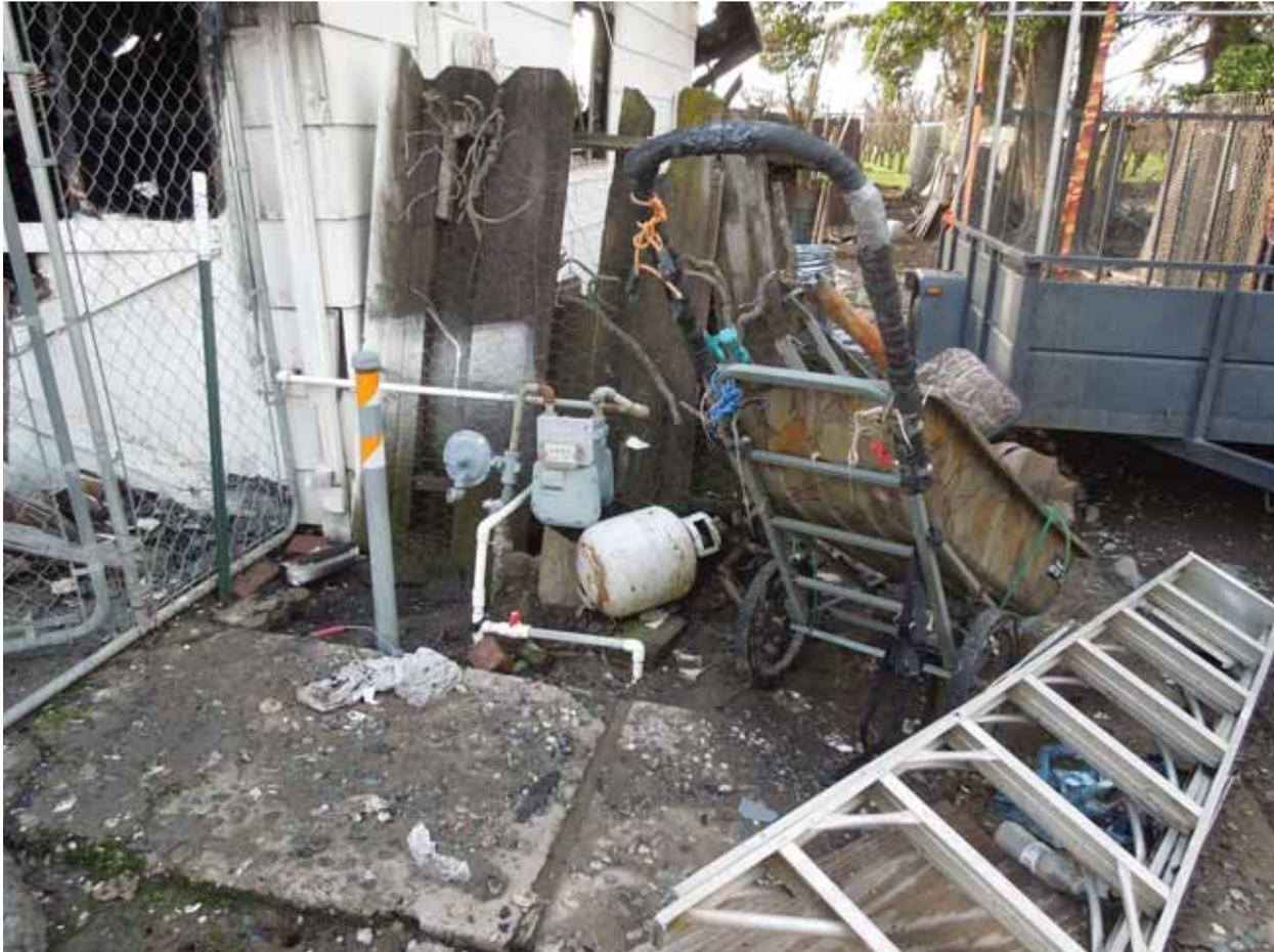
**Figure 5.** The meter set assembly (MSA)
