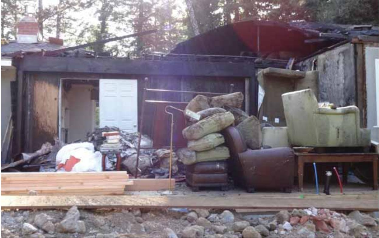
*Figure 4: The east side of the house; severely burned, with part of the roof burned away, or collapsed. The furniture had been removed for a remodeling project and is sitting on an outside porch.*
