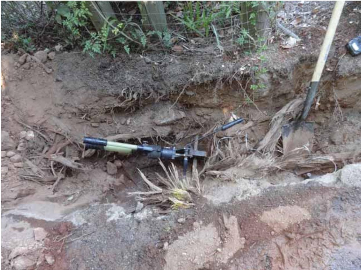
*Figure 13: The clamp squeezing the ¾-inch steel line shut at the front of the property.*
