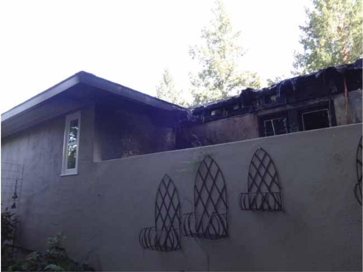
*Figure 2: The eaves above the gas meter and water heater burned away, exposing the interior of the attic. This picture is taken outside the small roofless enclosure, facing south.*
