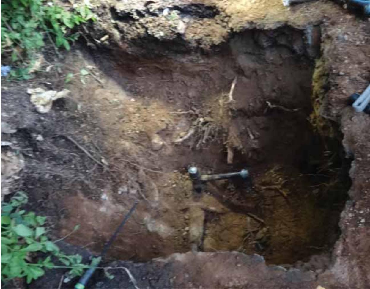
*Figure 14: The service line at the main; cut and capped.*
