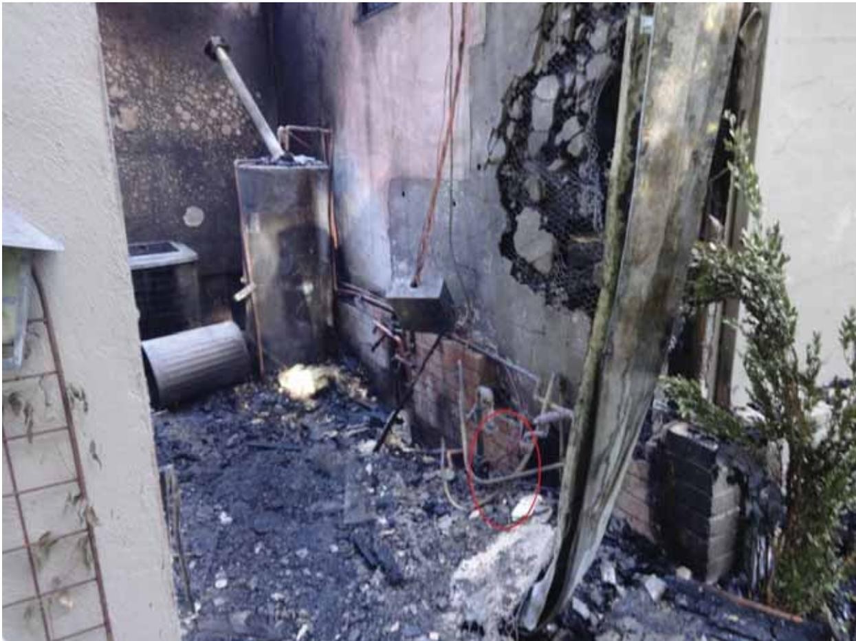
*Figure 1: The roofless enclosure that contained the gas meter, a water heater, an electrical service box, and an air conditioning unit. The red circle represents where the gas meter had been.*
