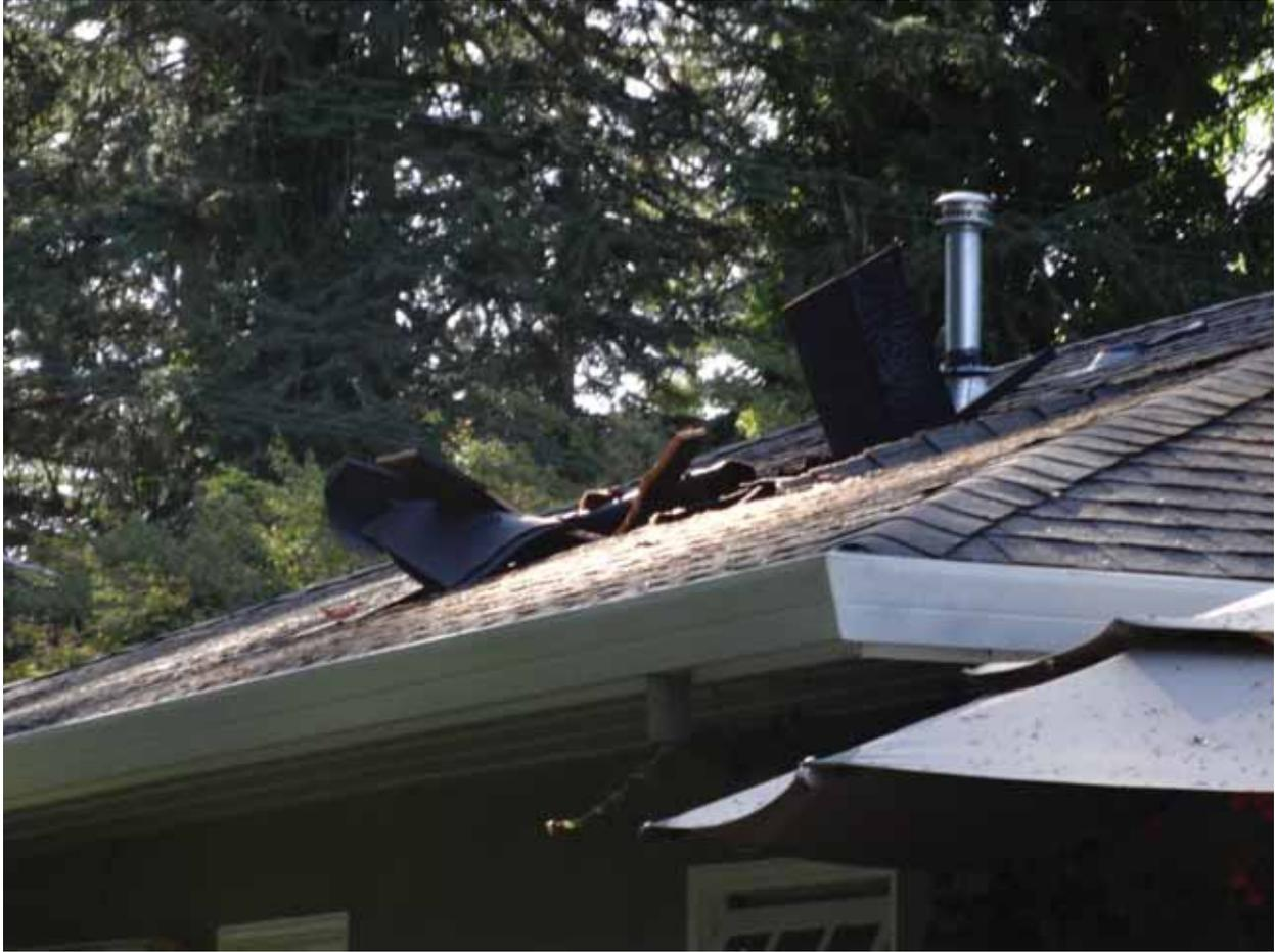
*Figure 7: A close-up of a damaged piece of roof on the southeast corner of the house.*
