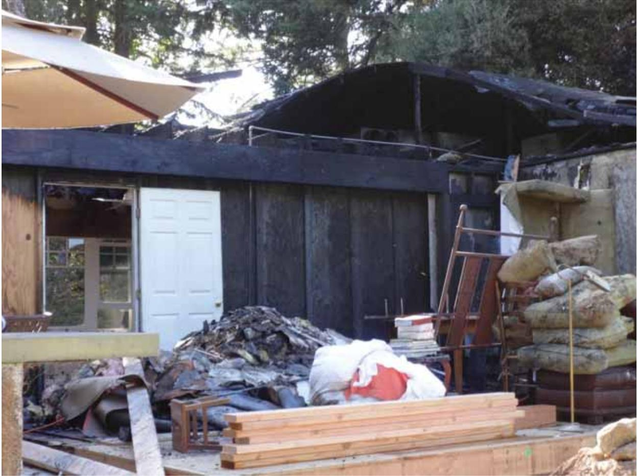
*Figure 5: A different angle of the east side of the house; severely burned, with part of the roof burned away, or collapsed. The furniture had been removed for a remodeling project and is sitting on an outside porch.*
