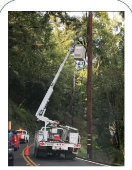
Figure 2 – Aerial fiber installation to provide broadband service in the CASF Nicasio Broadband Project, Western Marin County.
