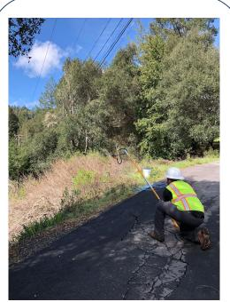
Figure 3 – Contractor launching throwline for a fiber pull in the CASF Nicasio Broadband Project, Western Marin County.
