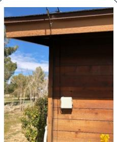
Figure 5 – Outdoor fiber enclosure at a residence in CASF Gigafy Phelan Project.
