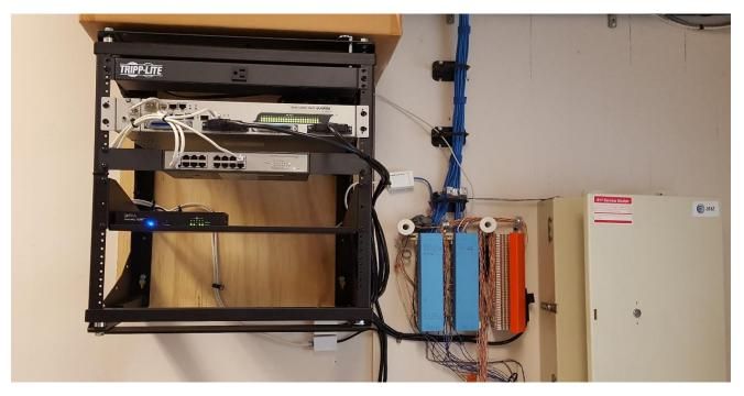
Figure 23: Village Park Apartments MDF Room with DSLAM, Firewall, Switch, Modem, and 66 Block
