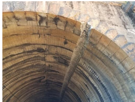
Groove in ceiling, UPRR Tunnel 34
