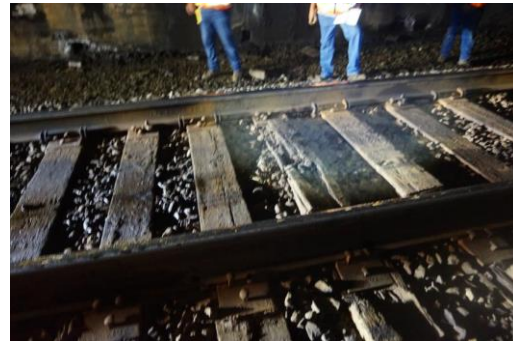
Loose spikes found in tunnel 33
