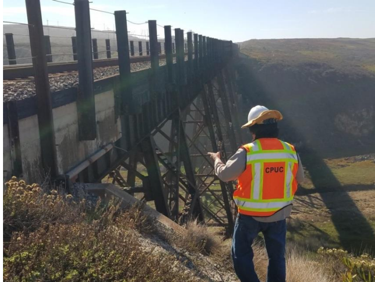
CPUC railroad safety bridge inspector looking over ballast deck bridge substructure for structural integrity and associated potential risks
