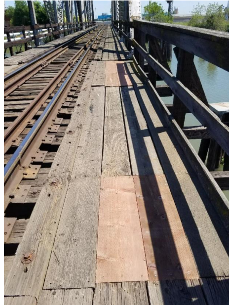
San Joaquin River bridge walkway after repair
