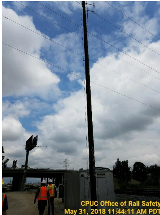
A CPUC inspector observed a UPRR PTC wayside installation and associated PTC radio equipment. PTC antennas are shown on the top of the pole.
