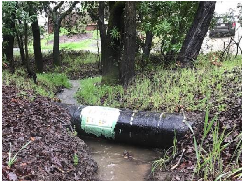
8 Figure 1-1: Picture of Exposed Segment of Pipeline 9 on Beechwood Drive trail in Lafayette 3
