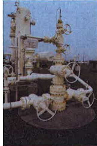
Typical Central Valley Gas Storage well
