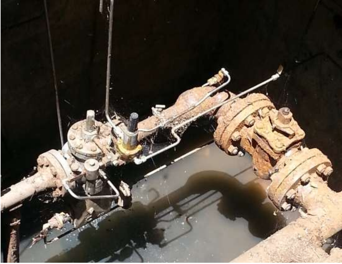
Figure 2. A photograph of corrosion at Regulator Station No. D-22.
