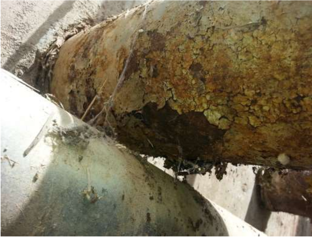
Figure 1. A photograph of corrosion at Regulator Station No. B-19.
