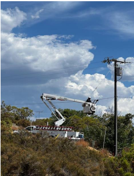
Figure 3: Anza Electric Coop placing fiber in the San Jacinto Mountain communities in Riverside County. This is a FTTH project that worked to install 3.7 linear miles of fiber on existing poles.
