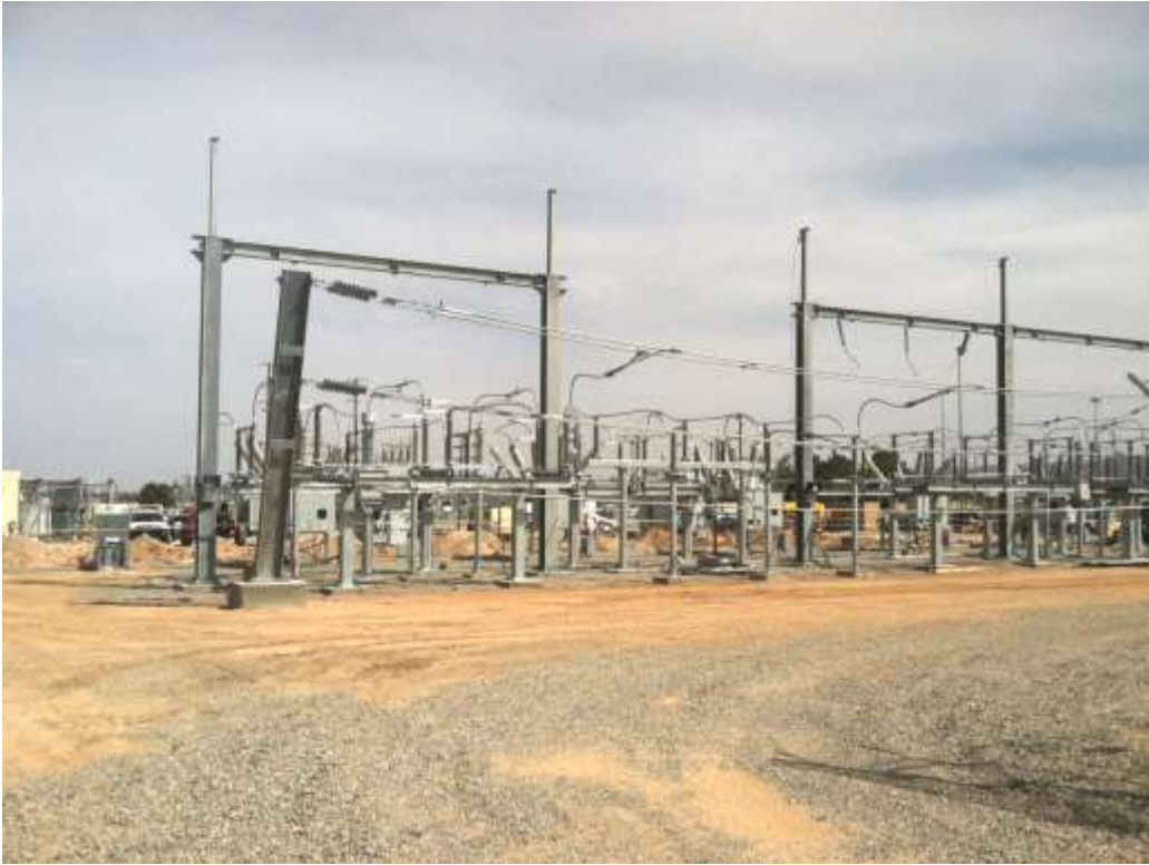
Figure 1 – The Downs Substation pad is approximately 60% complete. View southeast, 04/10/15.
