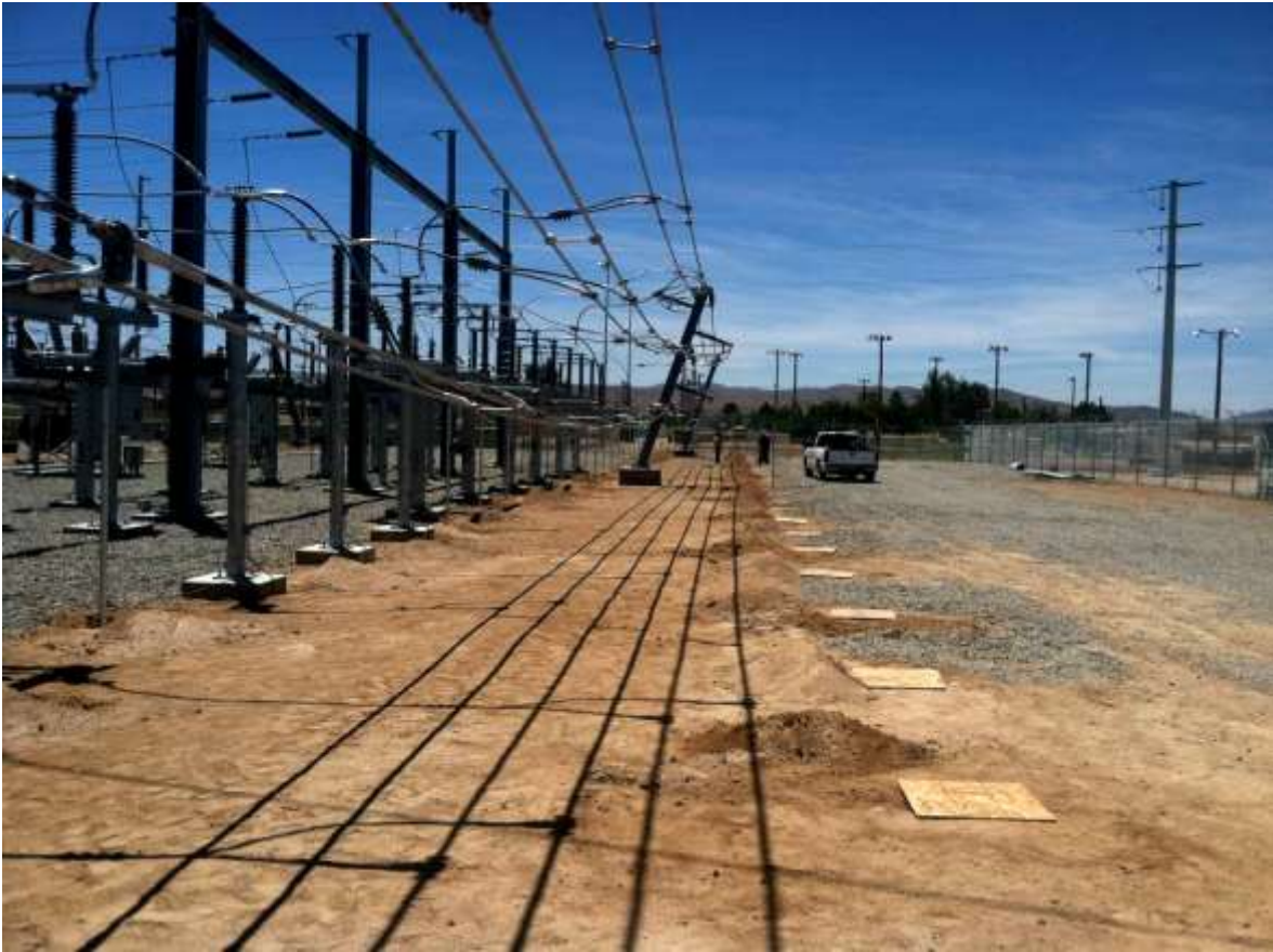
Figure 1 – Installation of interior fencing occurred during the subject period. View south, 5/29/15.
