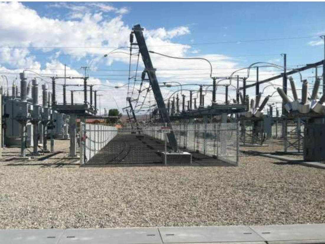
Figure 1 – Installation of interior fencing occurred during the subject period. View south,
