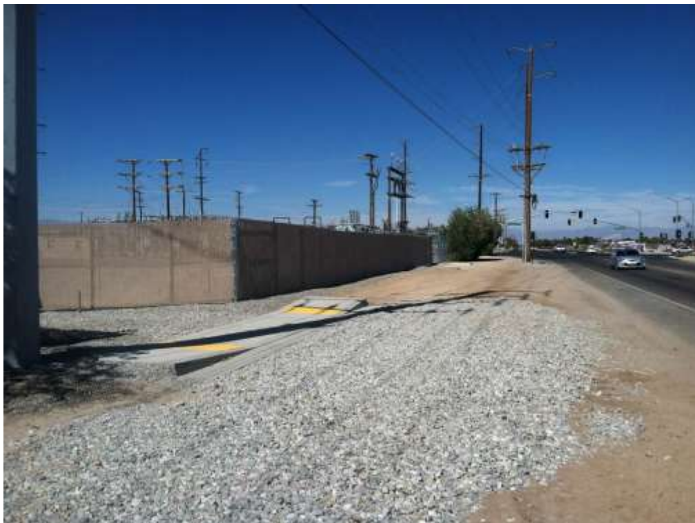
Figure 2 – Slated fencing can be seen shielding views of the substation along South Downs Street. View northwest.
