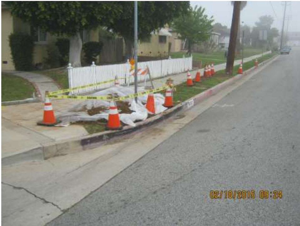
Looking N/NE from San Fernando Mission Blvd.
