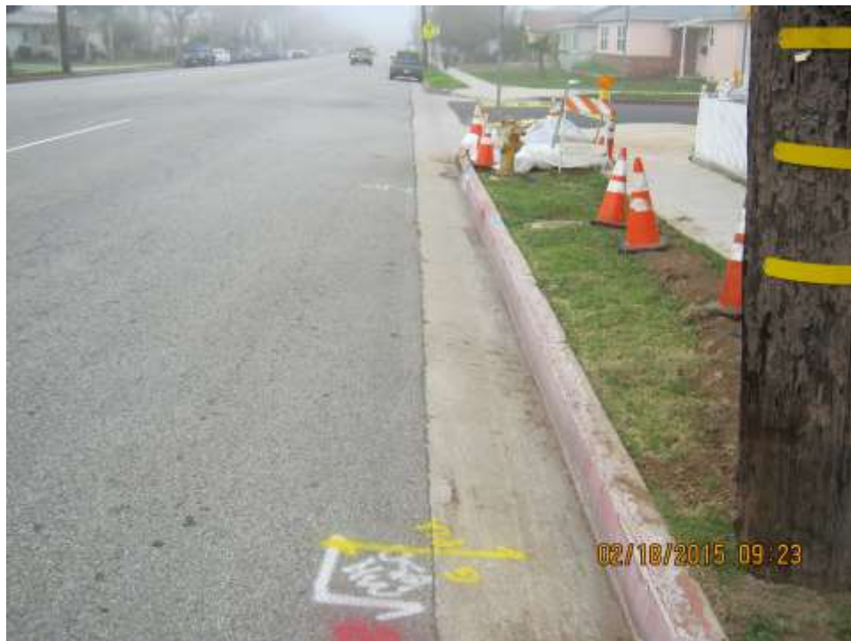
Looking W along San Fernando Mission Blvd.
