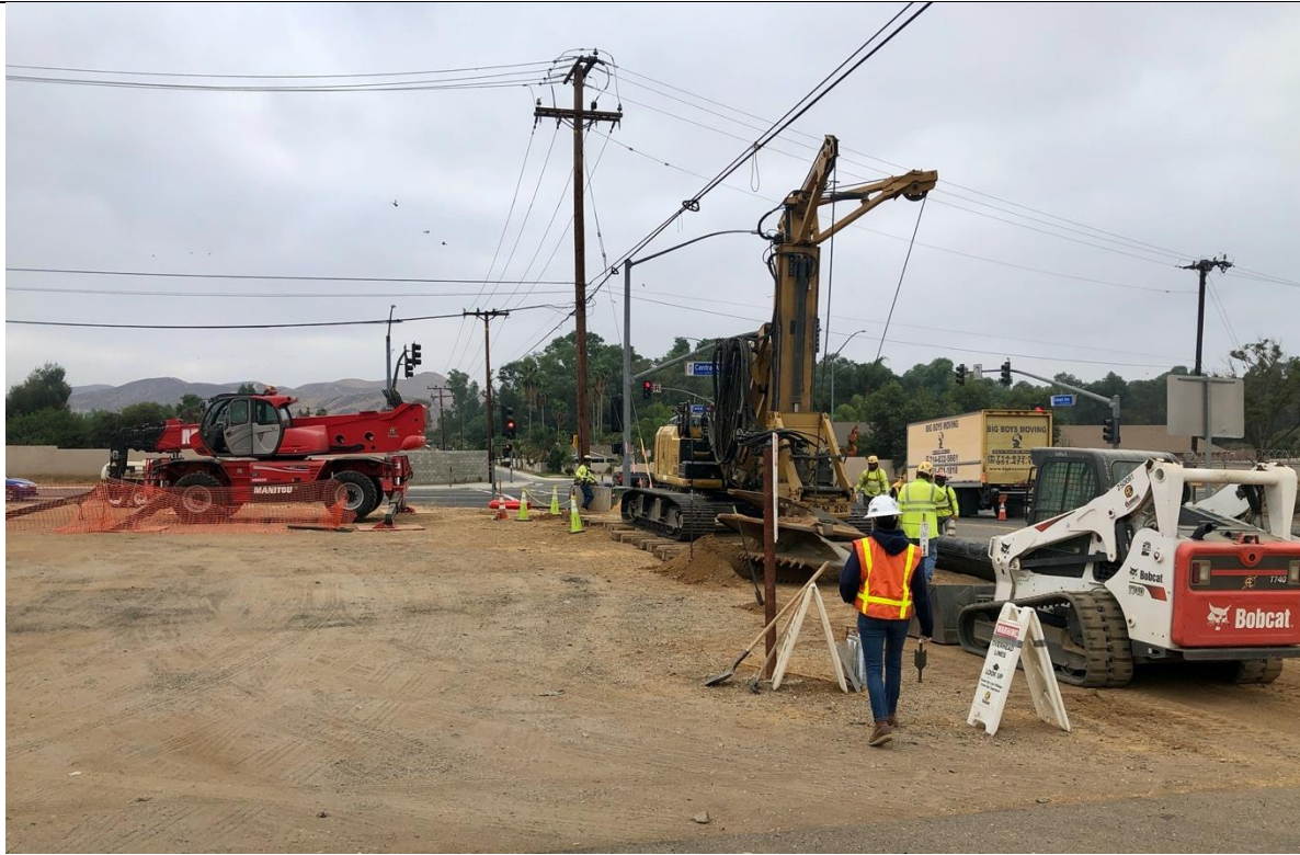
Photo 7 – Foundation work at Pole site 302E. Photo facing south
