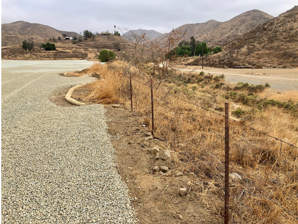
Photo 14 – Silt fencing and construction fencing will be installed around the entire yard. An ephemeral drainage exits just to the south of the yard. Photo facing east
