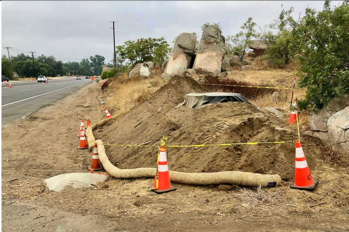
Photo 10 - Excavation site for wooden pole #212. Photo facing west
