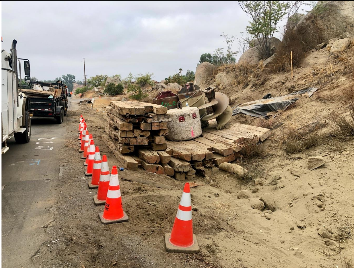
Photo 11 – Drilling operation to begin at pole site #213. Photo facing west
