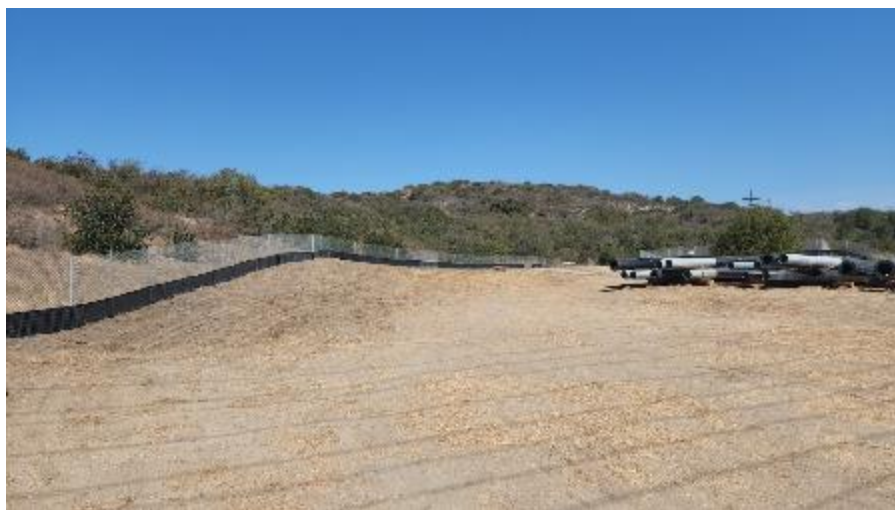
Photo 4: Northwestern-view of bare ground MPR-14 staging area.
