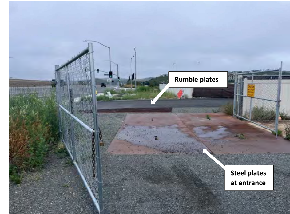
Photograph 1: View of the southwest corner and construction entrance of the Cow Camp Staging Area with previously placed Best Management Practices (BMPs) including rumble plates and flat plates that will be maintained throughout the course of the Project. Facing: Southwest.
