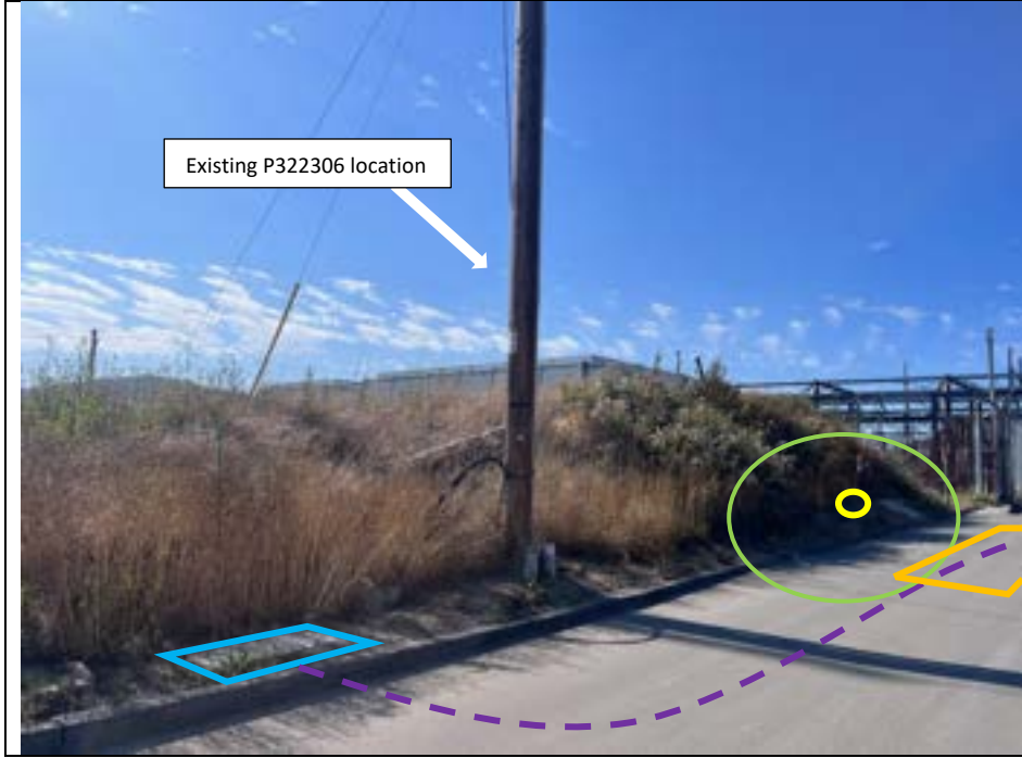
Photograph 3: Trenching (indicated by purple dashing) will occur within the existing road bed from the northern perimeter of the Talega Substation to the new handhole (orange polygon) that will be installed west of the MPR-21 work area (green circle). Trenching will then occur from the new handhole to the existing conduit (blue polygon) located 8 feet north of the existing P322306 location. Facing: Southeast.
