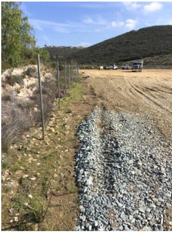
Caption Fence installation areas Stonebridge Yard
