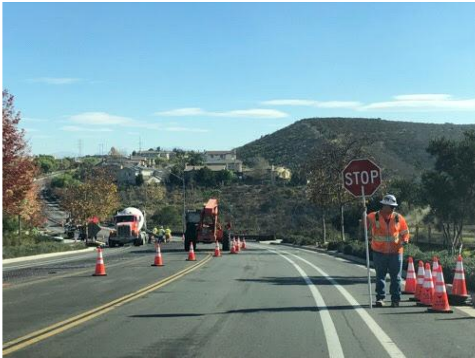
Caption Stonebridge Parkway cement work and traffic control.
