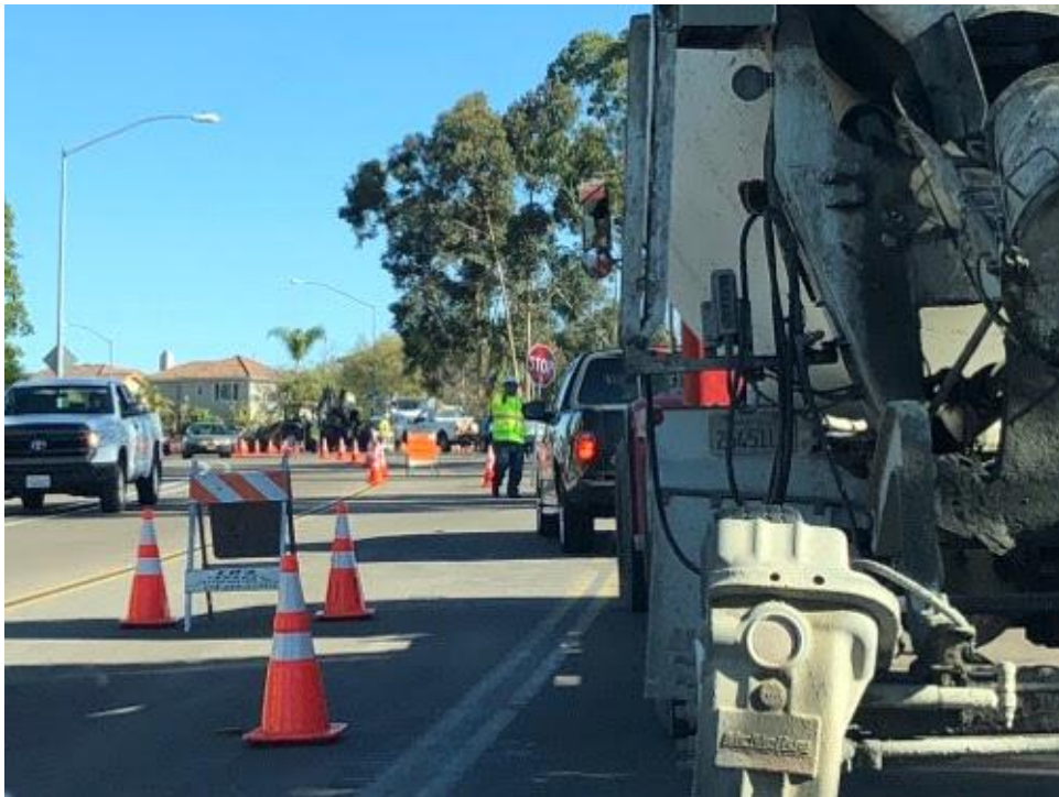
Caption Traffic control on Pomerado Road.
