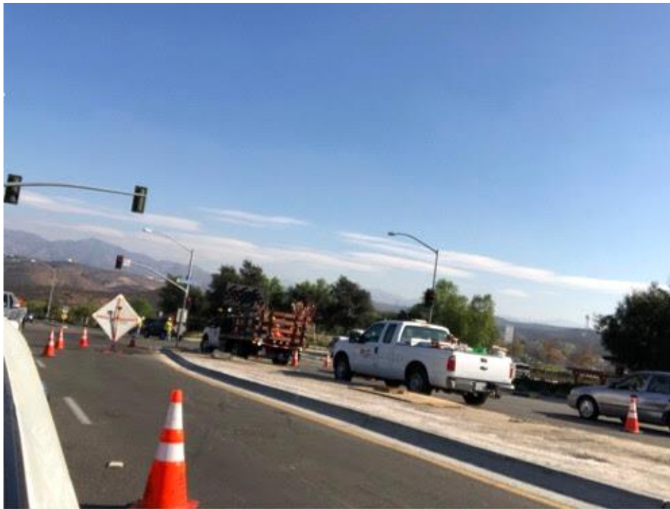
Caption Trench work at Pomerado Road just west of Stonebridge Parkway.
