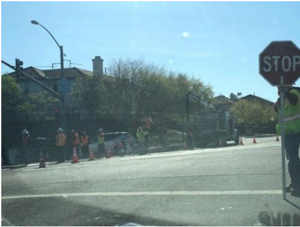
Caption Traffic control and cement work on Pomerado Road.
