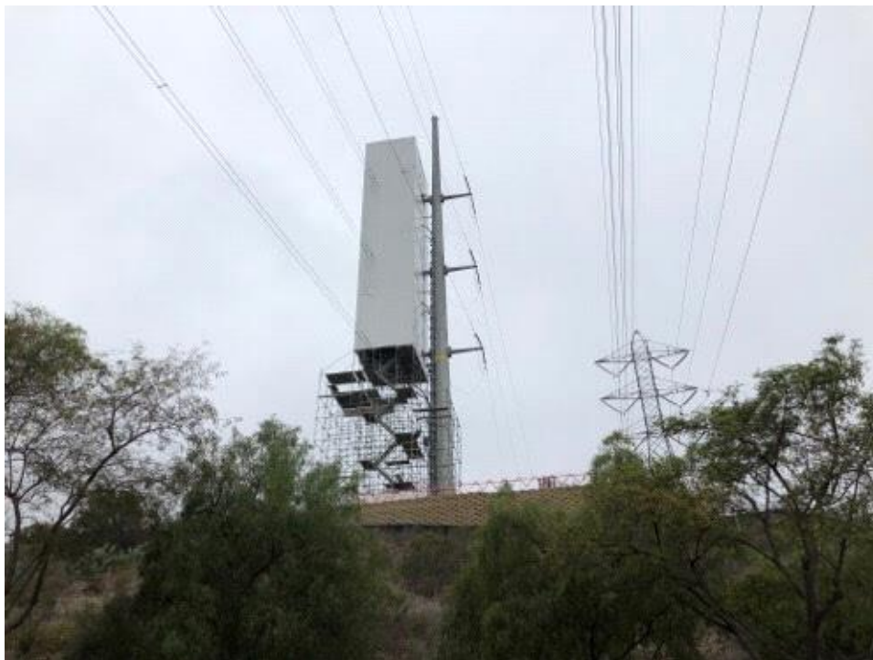
Caption P05 minor bolting QA/QC ongoing.
