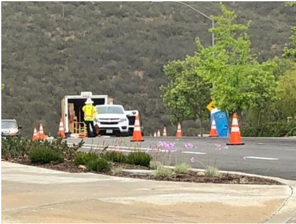
Caption Stonebridge Parkway vault work.
