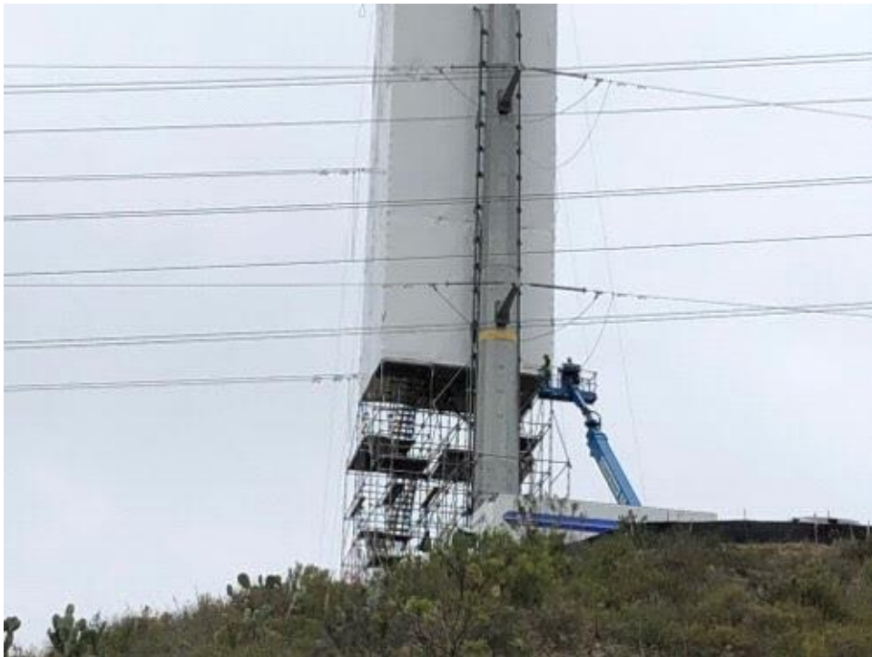
Caption P05 scaffolding work.
