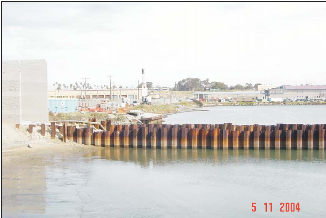
Looking east at the CPDMMB and Bulkhead.
