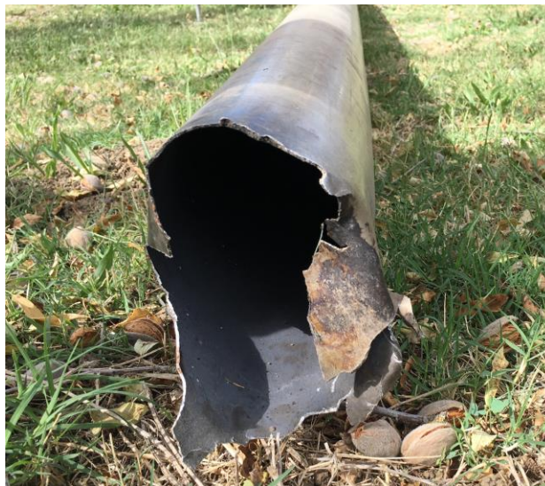
Figure 2. Remaining 26' section of irrigation pipe severed by electric contact.
