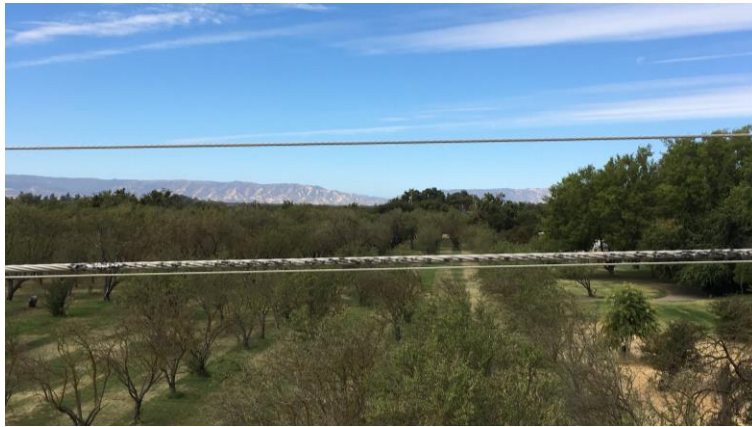
Figure 1. Arcing marks found on the conductor of Davis-1107, 12 kV circuit.
