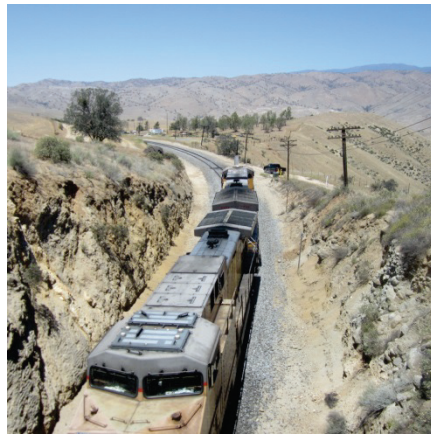
Westbound freight train exiting Tunnel #3 in Tehachapi Pass (Local Safety Hazard Site No.16)
