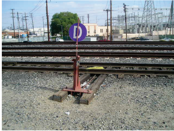
Derail not in derailing position, UP Alfalfa Lead, Alhambra Subdivision
